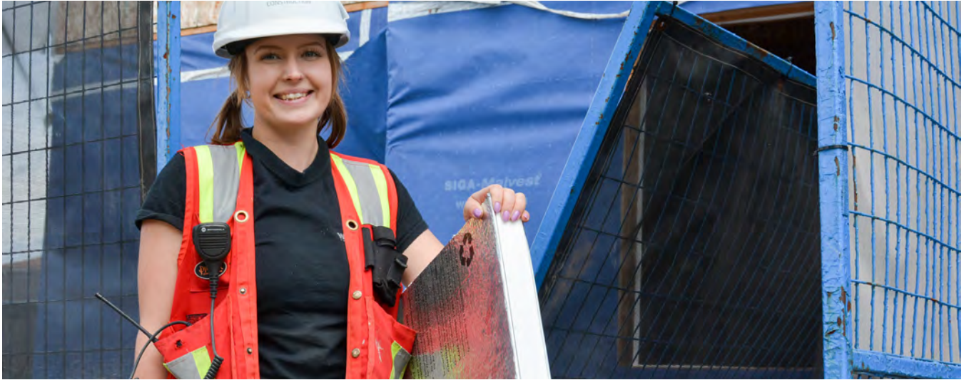
Passive House apartment building under construction in Vancouver, B.C. Photo: Stephen Hui
