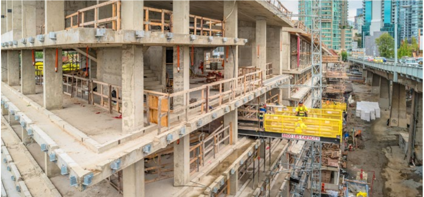
Construction workers work on a condo building in downtown Vancouver.
