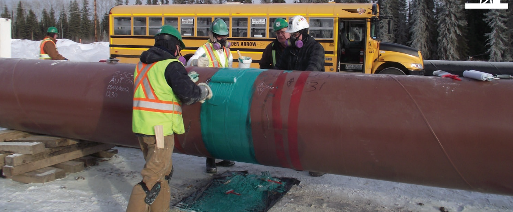
Albertan oil workers applying epoxy coating to a pipeline. Photo: jasonwoodhead23
